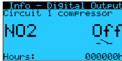
Figure_7.8: Digital Output Terminal NO2- Compressor 1
